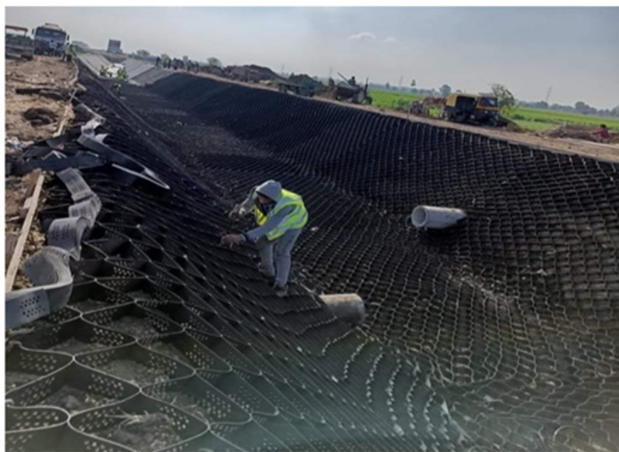
Figure 6: Geocell lining in the national project for canal lining - Egypt.
