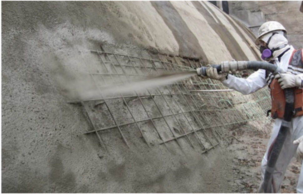
Figure 4: Lining by spraying concrete on the surfaces.
