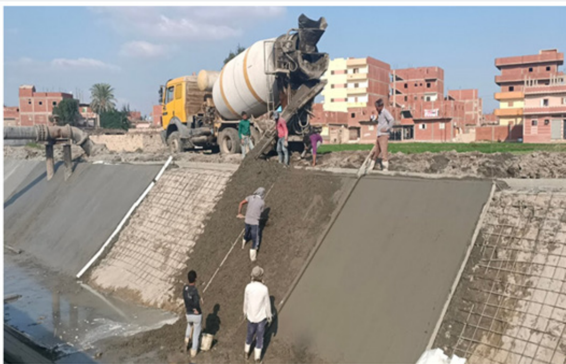
Figure 3: Lining by pouring concrete on the site.
