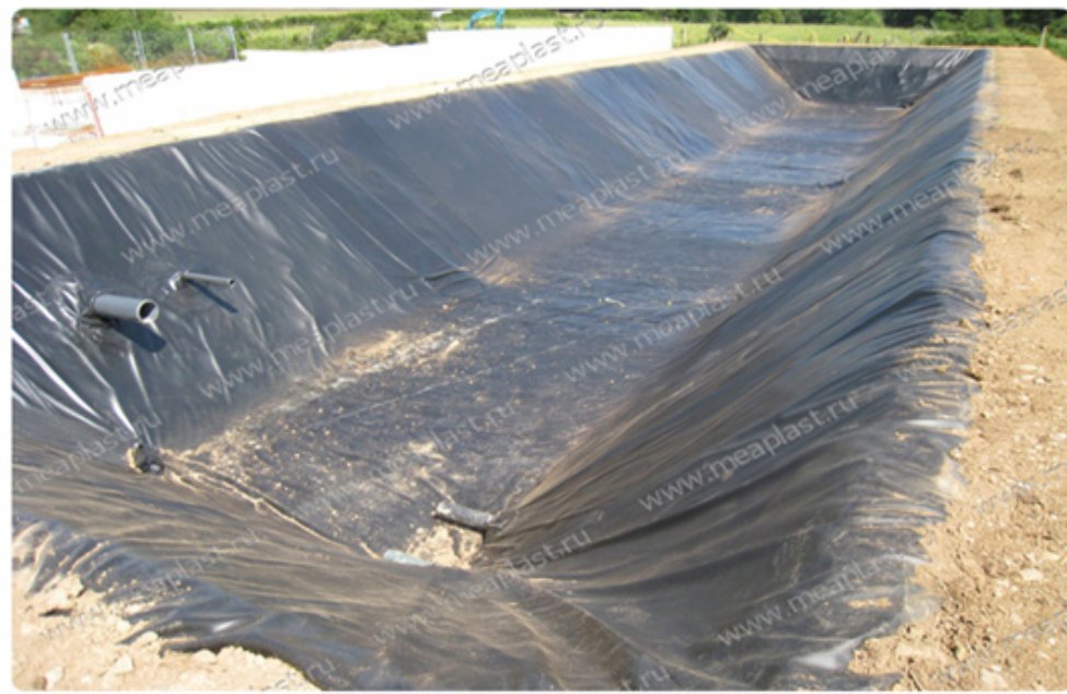
Figure 5: Lining with rubber membrane.
