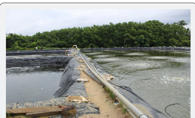
Figure 3: Ponds with lining and aeration.
