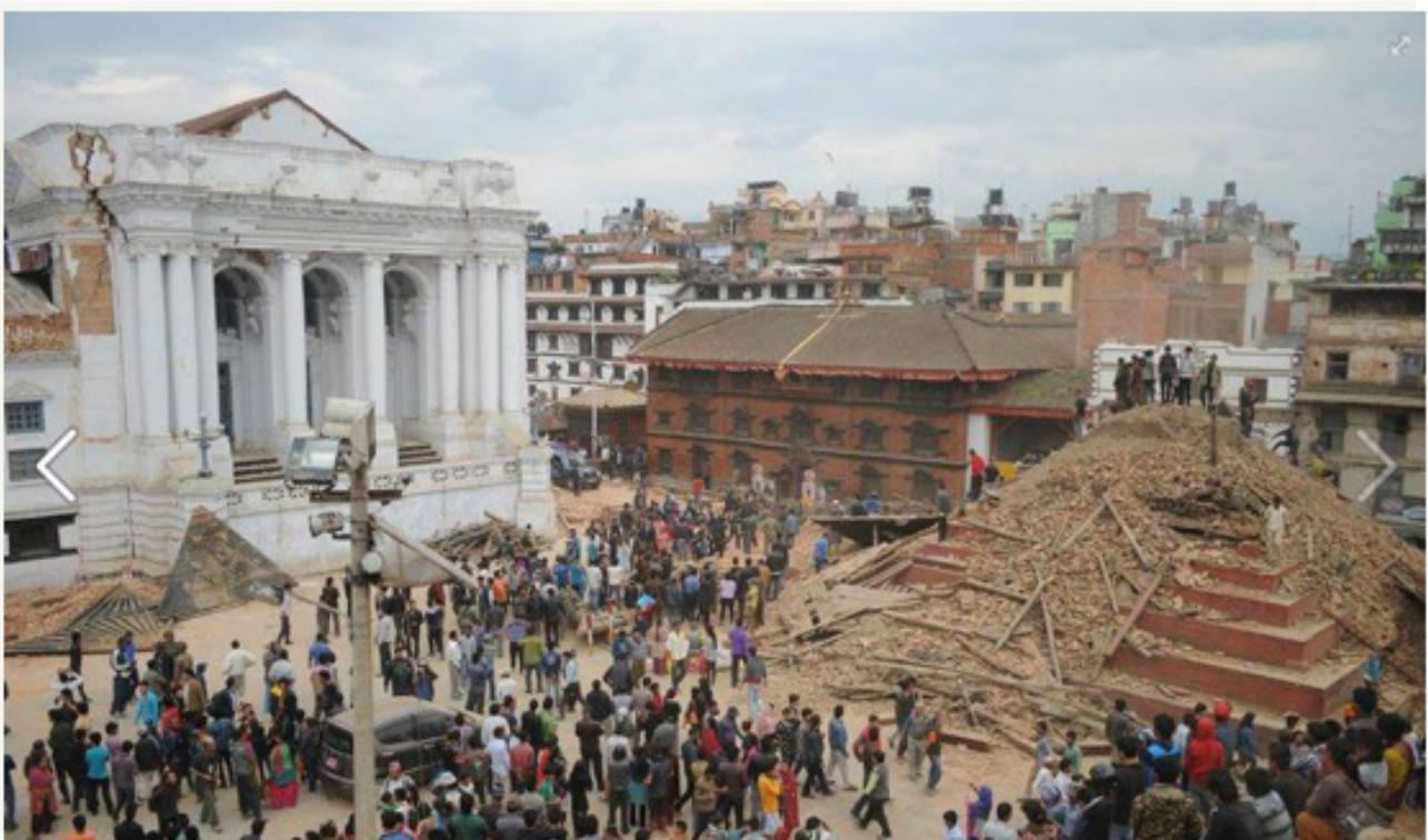
Figure 2: Damaged Kathmandu Durbar Square which is a Cultural Heritage.
