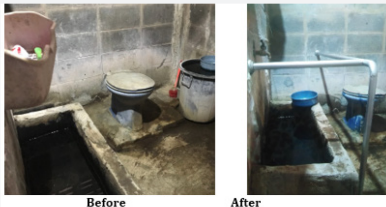
Figure 2: Installation of grab rails in the bathroom.
