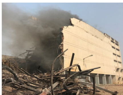
Figure 4: Another photograph taken during the incident of fire.
