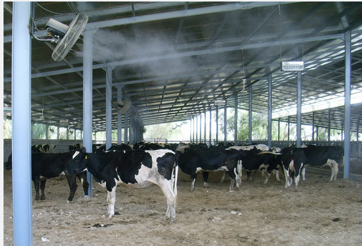
Figure 2: Misting fans can significantly reduce heat stress (Masterkool).
