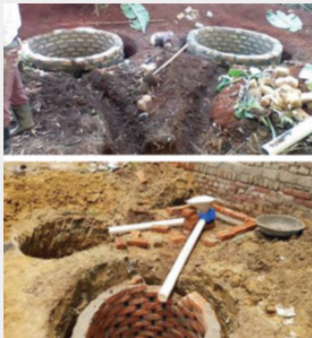
Figure 2: Layout of a double leach pour flush toilet on ground.
