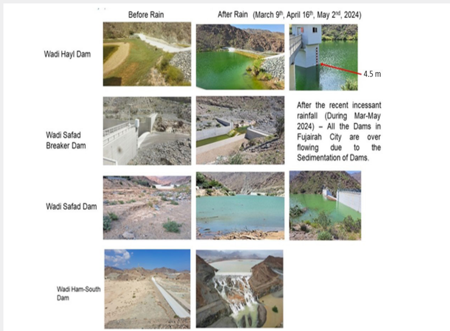
Figure 5: Water spilled over the Fujairah City Dams due to the Sedimentation upto the top of the Dam.
