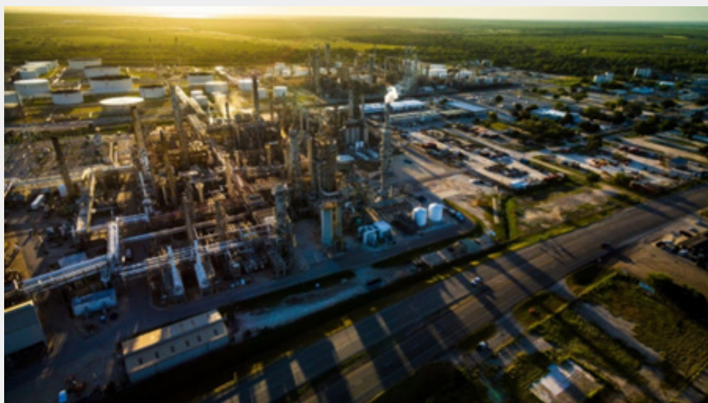
Figure 7: Aerial image for oil and gas expansions in our study area (Howard County, Texas).
