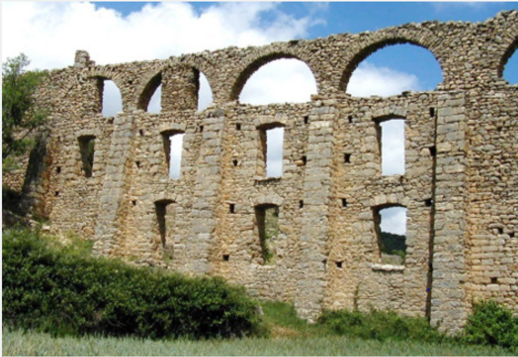
Figure 23: A section of the aqueduct bridge at Morella. Note the buttresses that were added later, and the window-like openings. Centering was used in the arches along the top. The arch supports were added later.
