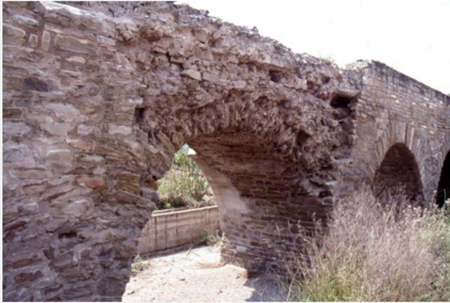
Figure 7: A view of a highly deteriorated portion of the aqueduct at Lodosa exposing various aspects of construction.
