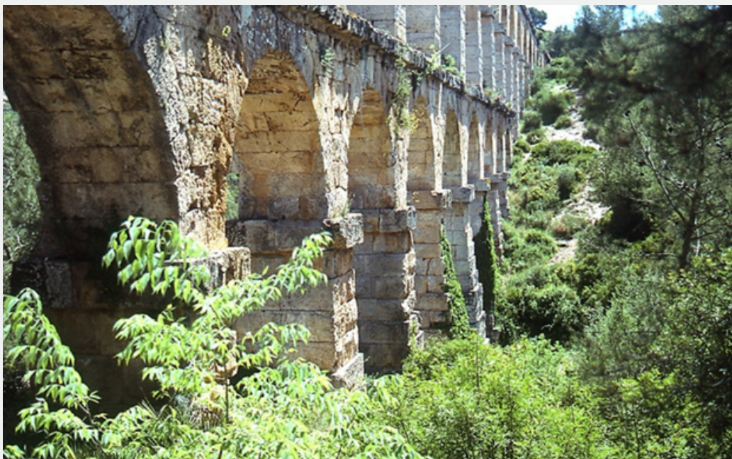
Figure 3: The elevated aqueduct in Tarragona. Note, the truncated pyramidal shape of the piers.
