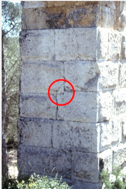
Figure 4: A close-up view of the joints between a few unique, rusticated rocks of the aqueduct bridge in Tarragona, showing that interchangeable parts had yet to be invented or adopted by the Romans.
