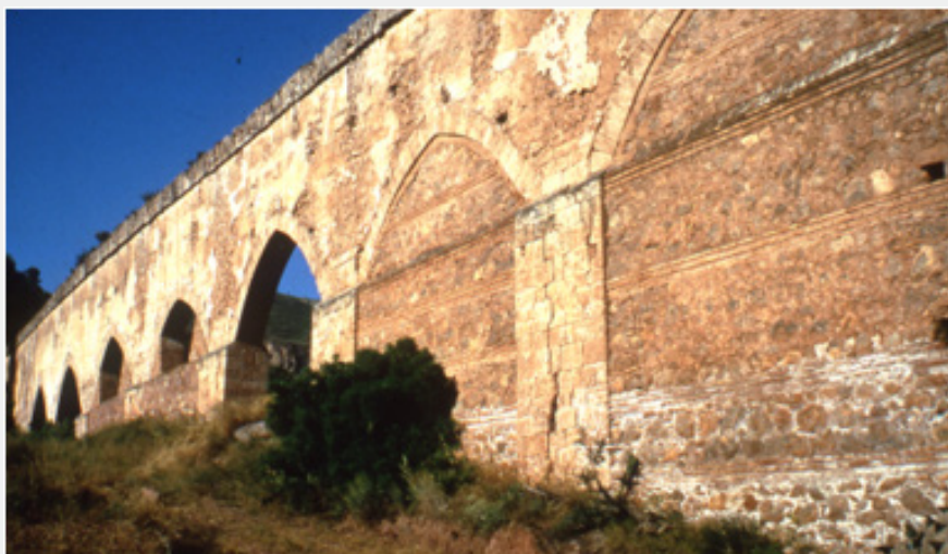
Figure 20: A view of the section of wall where the arches have been filled in. Remnants of a plaster coating are also visible. Image by the late Karl W. Butzer, used with permission of his wife.
