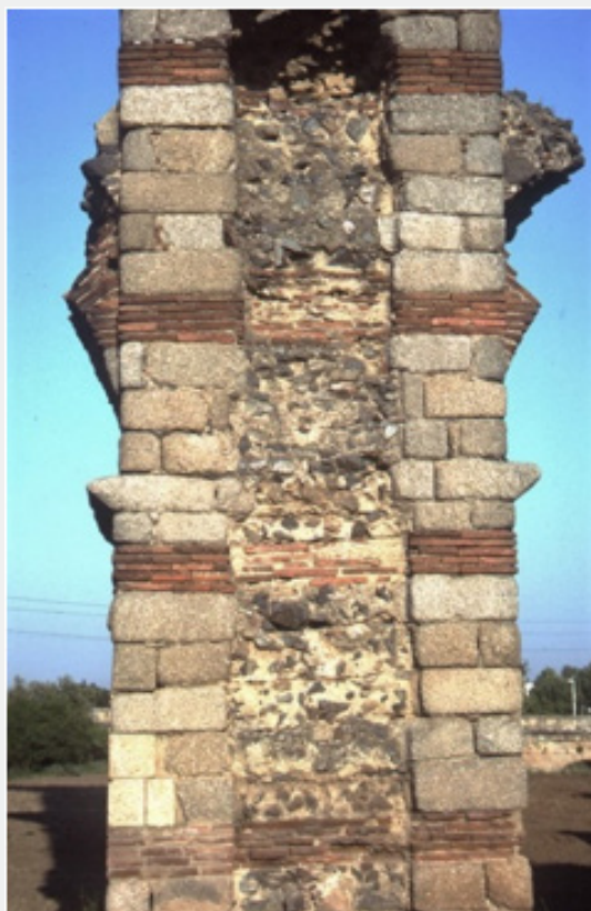
Figure 13: A close-up view of the composite construction of the aqueduct bridge in Mérida. The buttress added after initial construction no longer exists.
