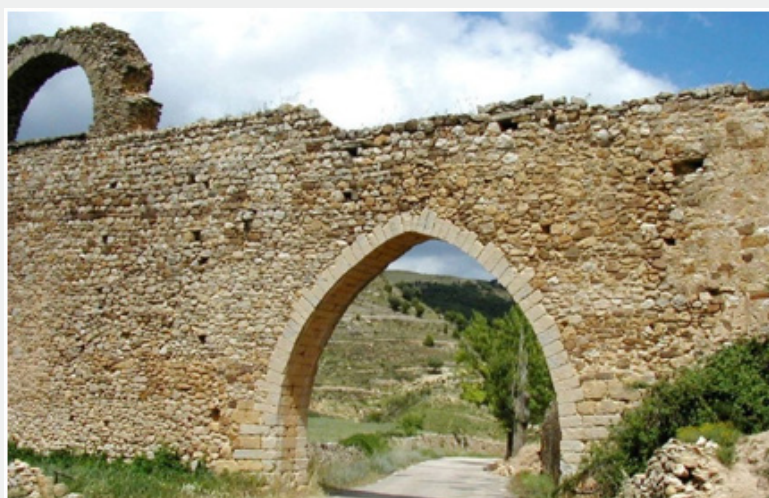
Figure 22: A Gothic arch in the Morella aqueduct. Note the structure here is principally a rock wall, and note the rubble on the right.
