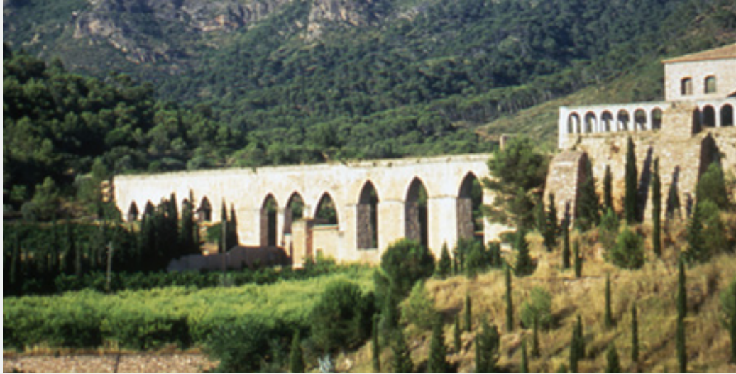
Figure 18: The elevated aqueduct at Puerta Coeli. Note the various thicknesses of piers and the variable heights of the arches. Image by the late Karl W. Butzer, used with permission of his wife.
