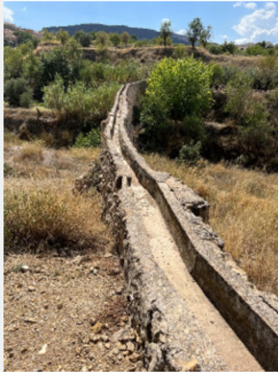
Figure 27: A view along the top of the Biar aqueduct. Note the narrowness of the elevated section, its waviness, and buttresses.
