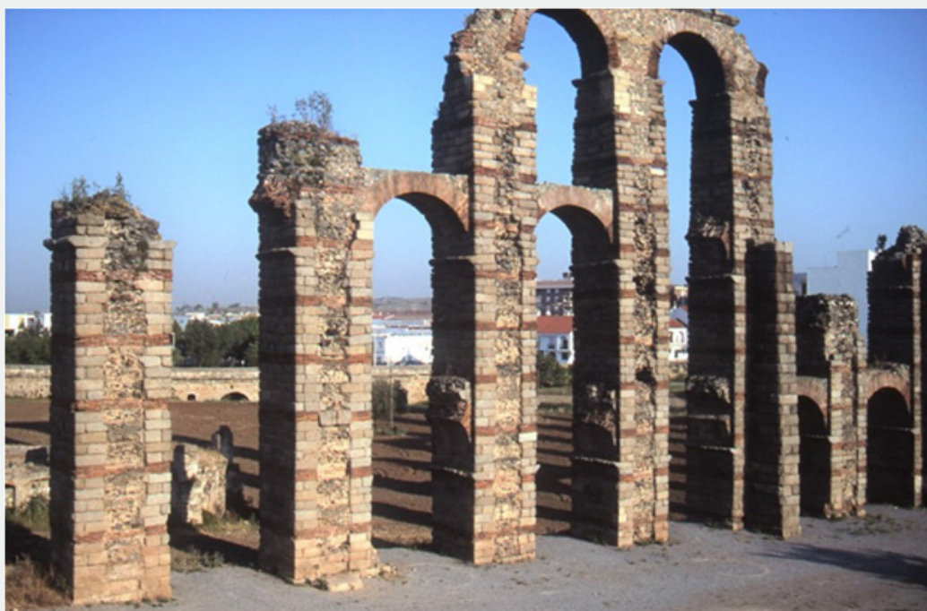
Figure 12: The elevated aqueduct of las Milagros in Mérida, Extremadura. Note the buttress on the fifth pier from the left, and the exposed cores of the first four piers where the buttresses no longer stand.
