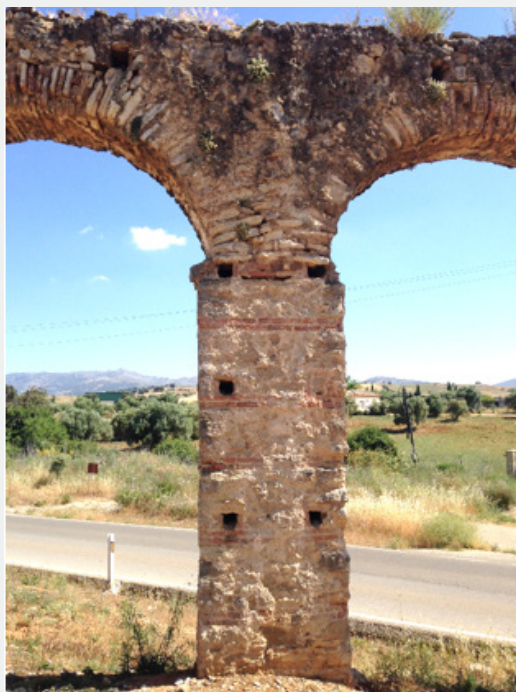
Figure 11: A close-up view of the opus incertum construction of the aqueduct bridge near Ronda.
