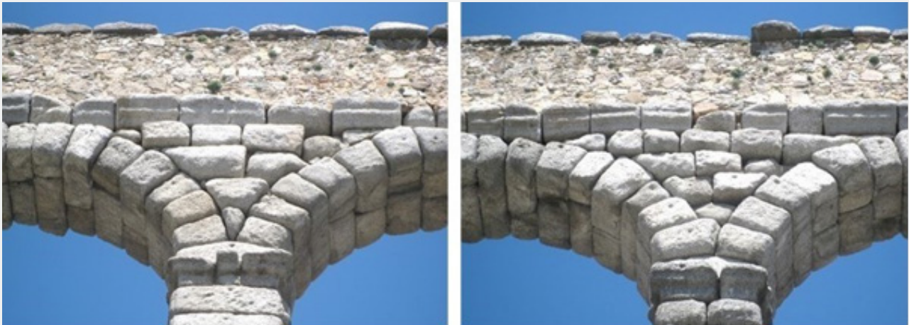
Figure 2: A view of two adjacent spandrels on the aqueduct bridge in Segovia. Note the unique shape of each rock.
