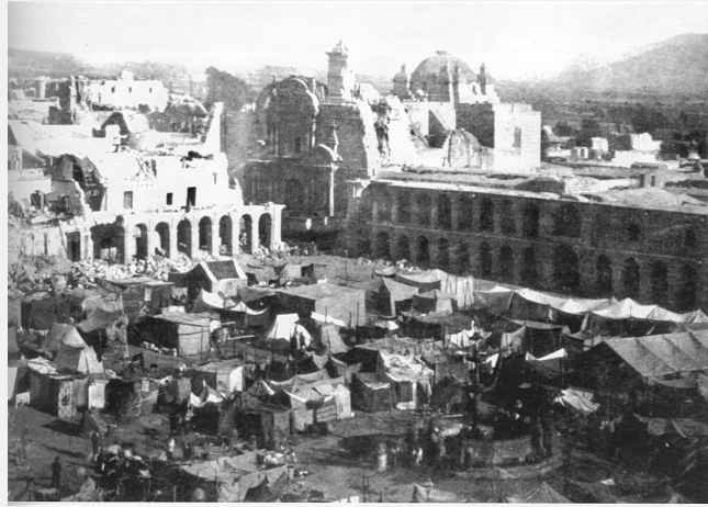
Figure 2: State of the arcades after the earthquake of 1868 [10].
