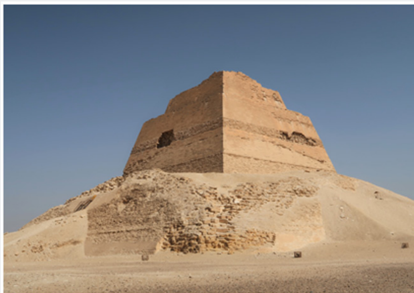
Figure 5: The pyramid of Meydûm from the north-west with the pyramid mantle exposed.
