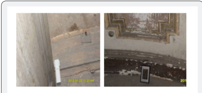
Figure 3: The Hygrometer which used for measuring humidity and temperature in and out of El Sakakeny palaces.
