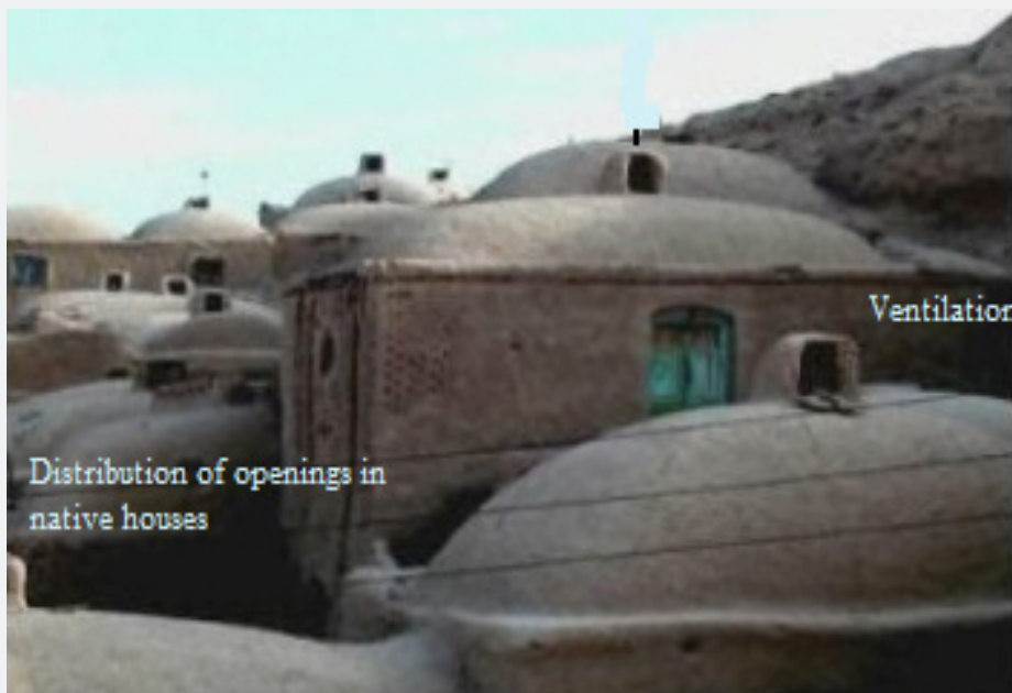
Figure 7: One side ventilator (Kolak) in Sistan [12].
