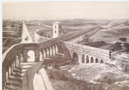
Figure 1: The Anio Novus and the Claudia aqueducts (left foreground) of Rome restored in a single structure and the Marcia, Tepula, and Julia (right). Painting by Zeno Diemer, courtesy of Deutsches Museum, Munich [1].
