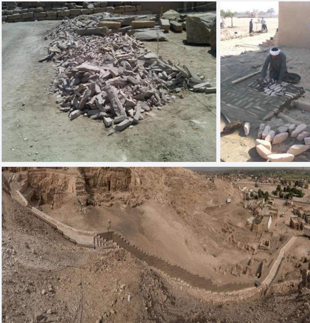
Figure 3: Use of stone scrap material to build walkways and stairways with mud brick buttresses.
