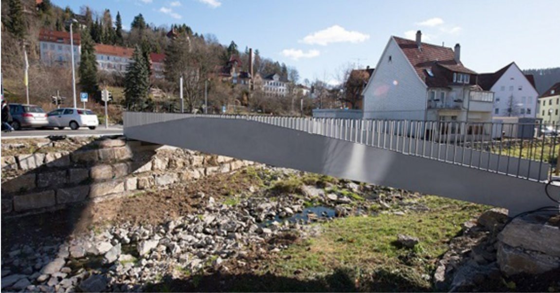
Figure 3: Pedestrian Bridge in Germany, the city Albstadt-Ebingen constructed as the very first experiment of concrete on the basis of carbon fiber (Carbonbeton), 2016.
