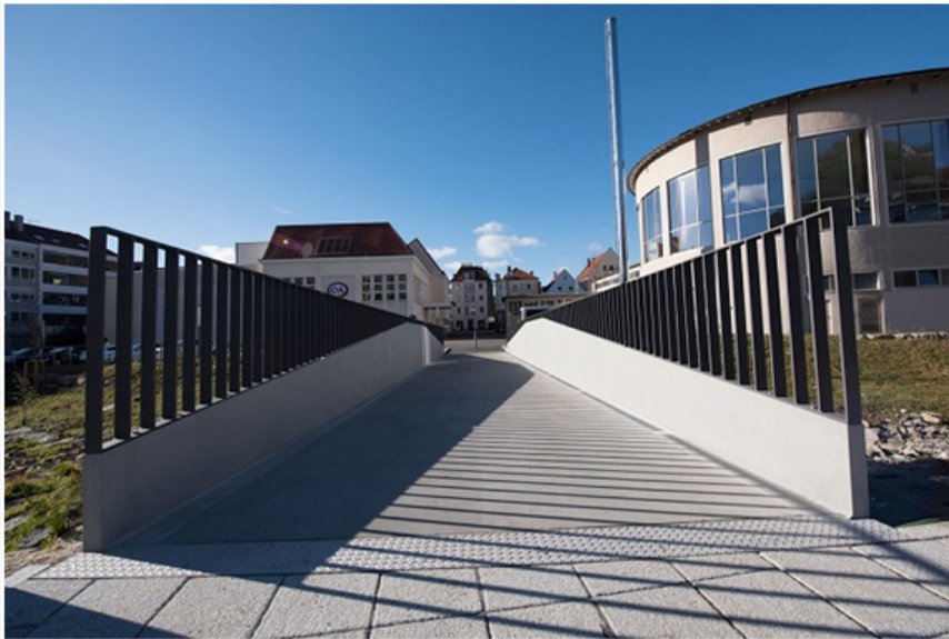
Figure 4: Pedestrian Bridge in Germany, the city of Albstadt-Ebingen, the first in Western Europe experiment from carbon fiber, 2016.
