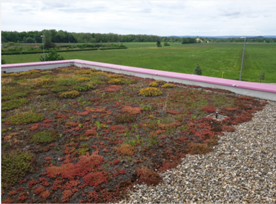
Figure 6: Sedum sp. the vegetation roof changes colour towards red shades in summer due to the formation of anthocyanins in the leaves.
