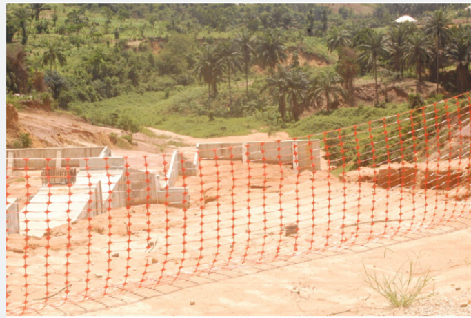
Plate 4: Gully control structure at Anua Offot, Uyo urban, Akwa Ibom State, Nigeria.
