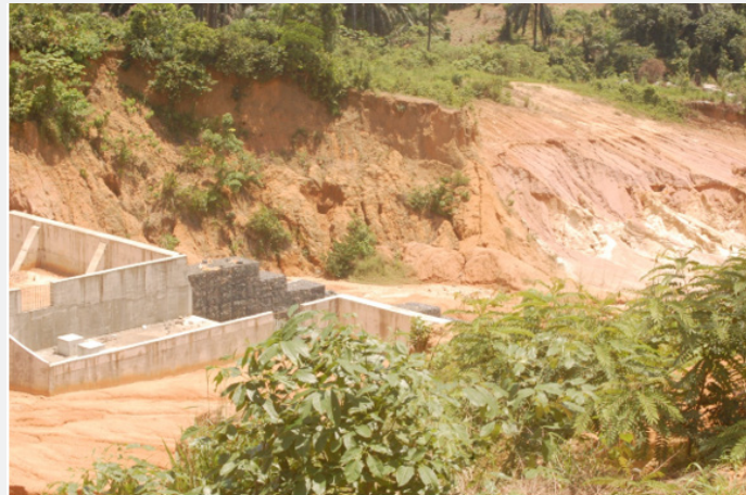
Plate 5: Extension of Anua gullies and the level of intervention.
