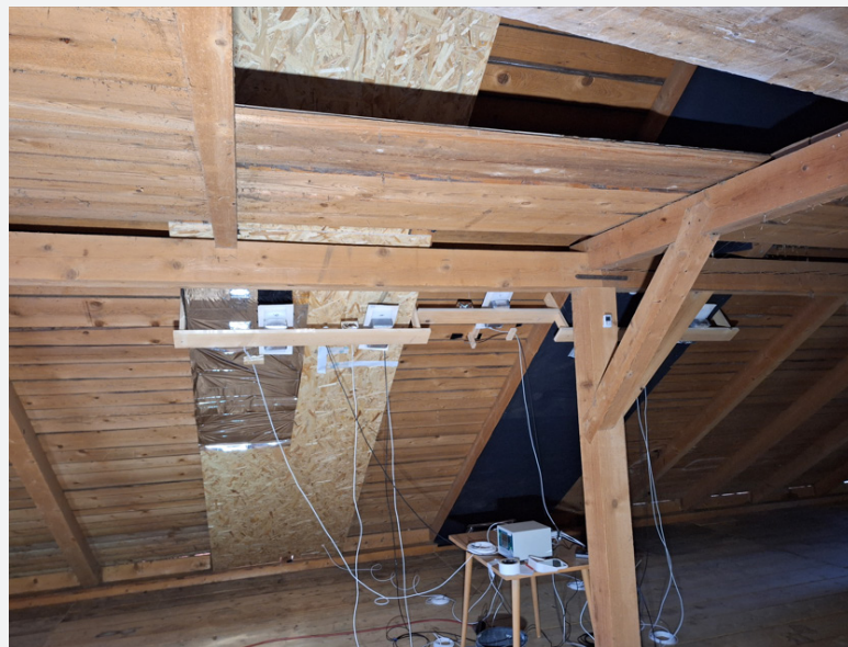
Figure 1: Rafter fields with OSB planking left (partly aluminum coated) and underlay membrane right.
