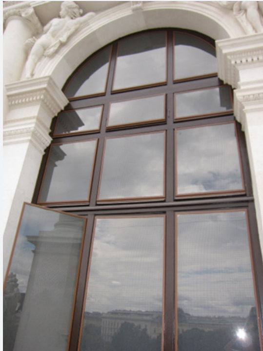
Figure 5: Shading elements on a window of the "Neue Burg" in Vienna, Austria.
