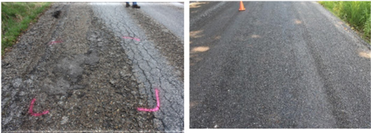
Figure 2: Noble County IN, Roadway Before and After Partial Depth Reclamation and Stabilization.
