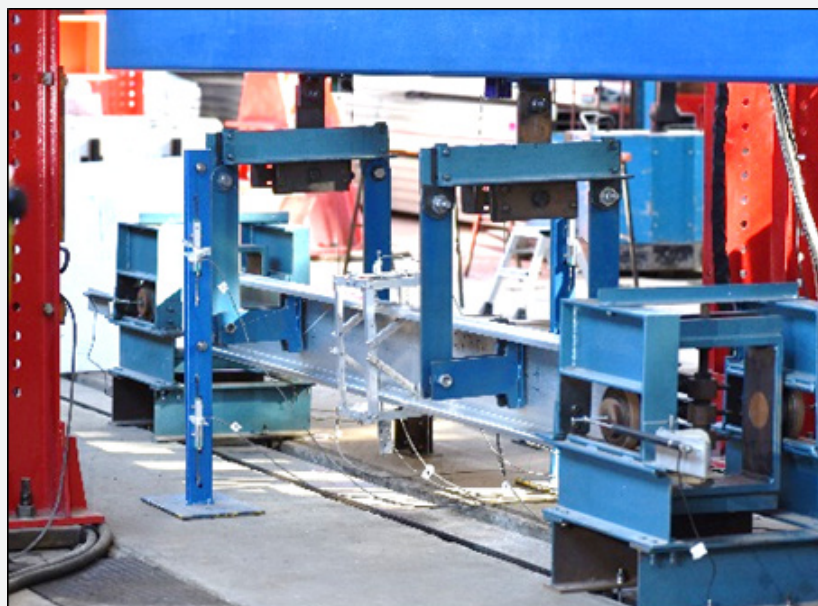
Figure 3: The test rig for downturn lip channel section beams.
