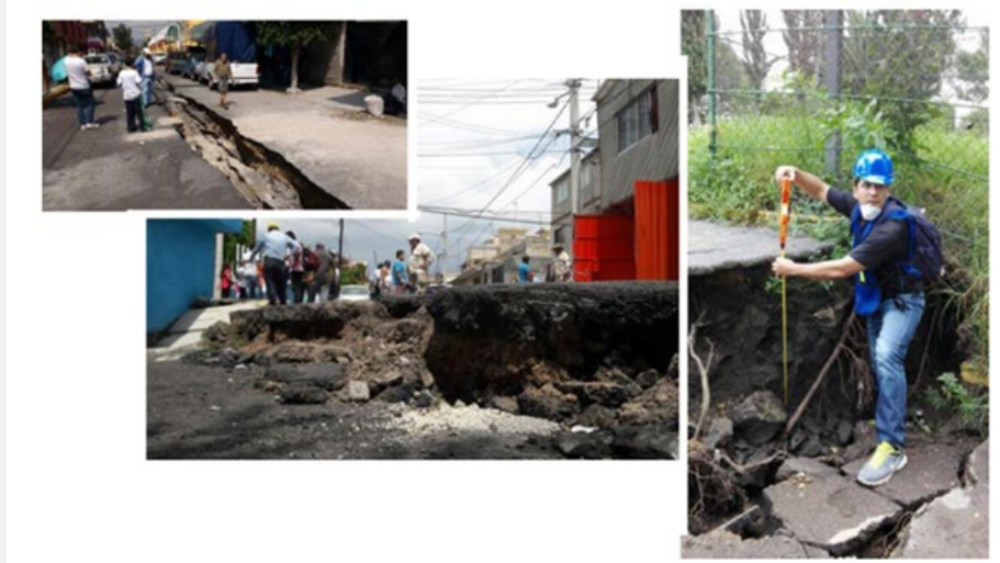
Figure 1: Effects of subsidence in the Transition Zone in Mexico City, sudden manifestations that occurred during the earthquake of the September 19 th , 2017 (M7.1).
