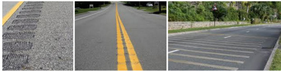
Figure 1: Three types of rumble strips - shoulder, centerline and transverse (TRS).
