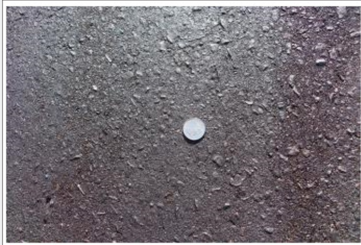
Figure 9: Asphalt Surface Texture Compacted with the AMIR.
