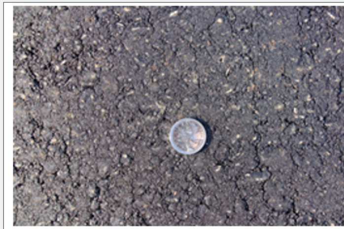
Figure 10: Asphalt Surface Texture Compacted with Conventional Rollers.
