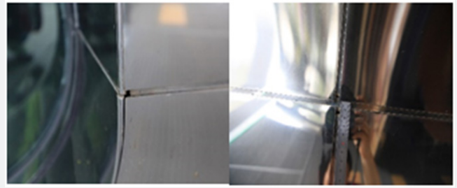
Figure 2 (b): Pictures of J Museum. Defective Fabrication Examples [15].
