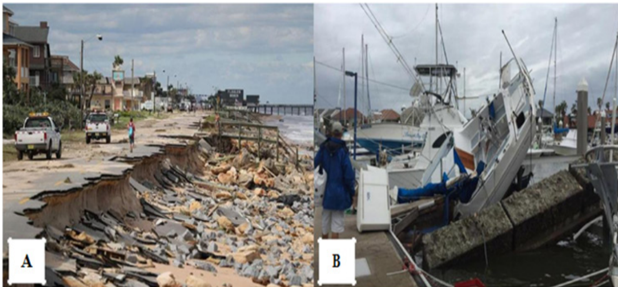
Figure 2: (A) Extensive Damage of Road after Storm Surge (Hurricane Jeanne, 2004), (B) Port Damaged after Storm Surge (Hurricane Irma, 2017) (NHC, U.S).
