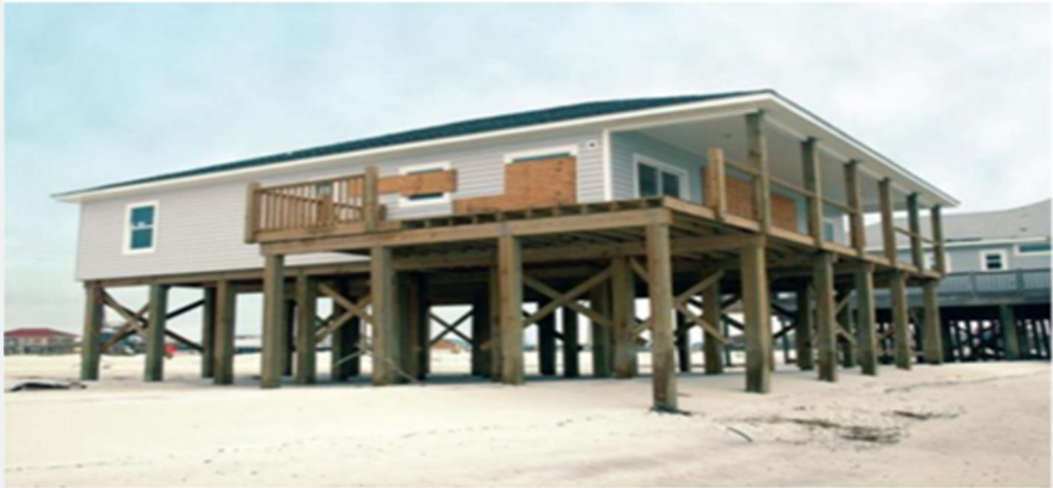
Figure 5: Elevated Buildings (FEMA 549, Hurricane Katrina in the Gulf Coast).
