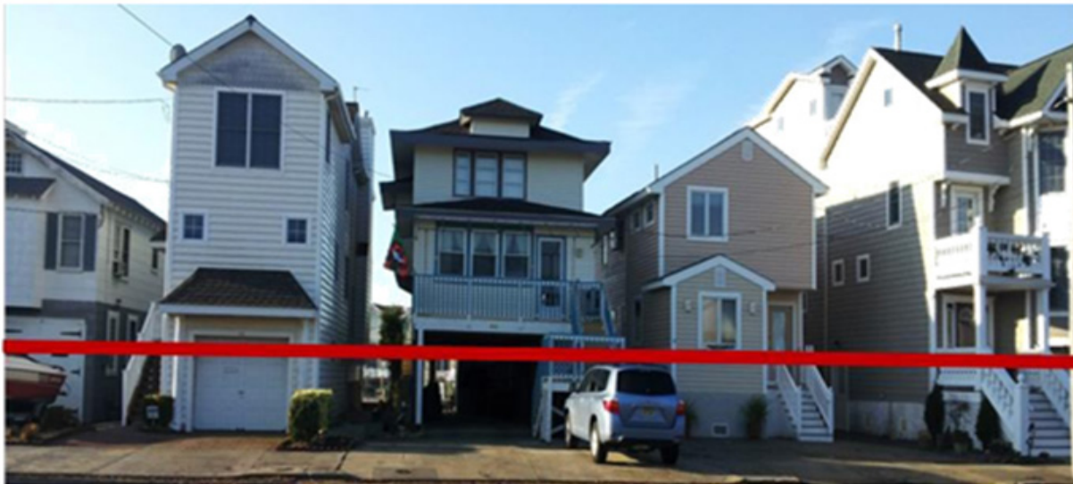
Figure 4: Houses with Different First Floor Elevations and Foundation Type Red Line shows the Level of Storm Surge (AIR Worldwide 2015, Hurricane Sandy).
