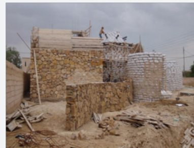
Figure 4: Qusayr Al-Jawasreh construction Watanabe [11].
