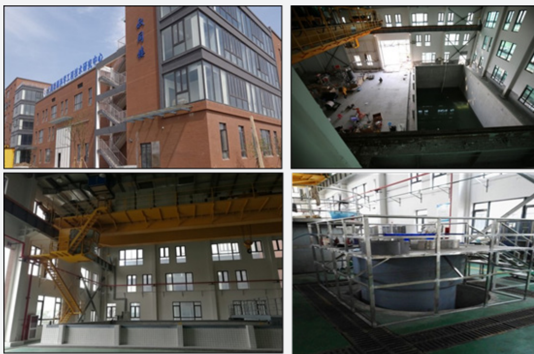
Figure 7: “Shutong building” for the assembly of submersibles. Its total space is 2600 m 2 , it has a crane with a capacity of 30 tons, a small open water tank with a size of 20m (length)×10m (width)×7m (depth) and four pressure chambers whose maximum test pressure from 140 MPa to 180 MPa.
