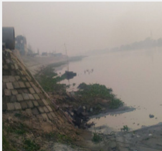
Figure 8: Discharge of untreated effluents in Dhaleshwri river.
