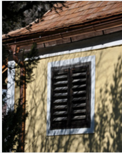
Figure 1: Wooden shutters - a proven low-tech approach for window shading with high aesthetic value.
