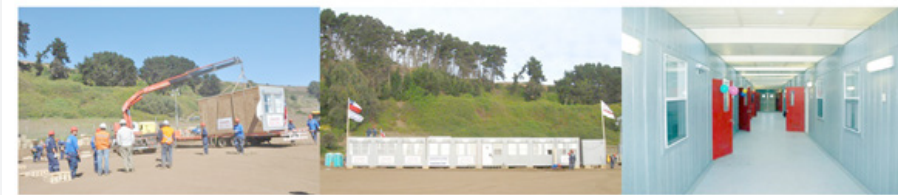
Figure 5: Modular Illoca School, the installation process.
