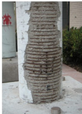
Figure 6: Typical examples for the failure of concrete. Compression failure (left) and buckling failure (right). [15].
