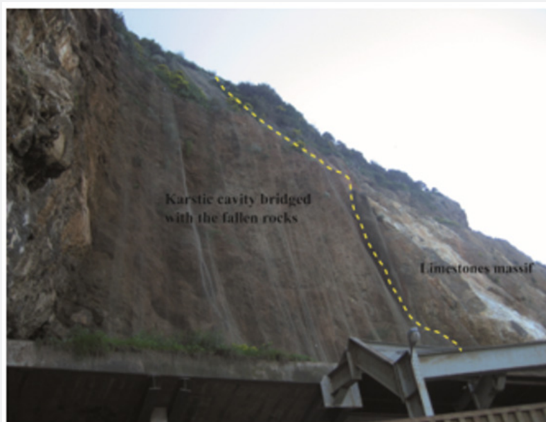
Figure 10: Breaking surface (S) cleared by the rock fall in the calcareous slope and destabilization of the fallen rocks of karstic cavity.
