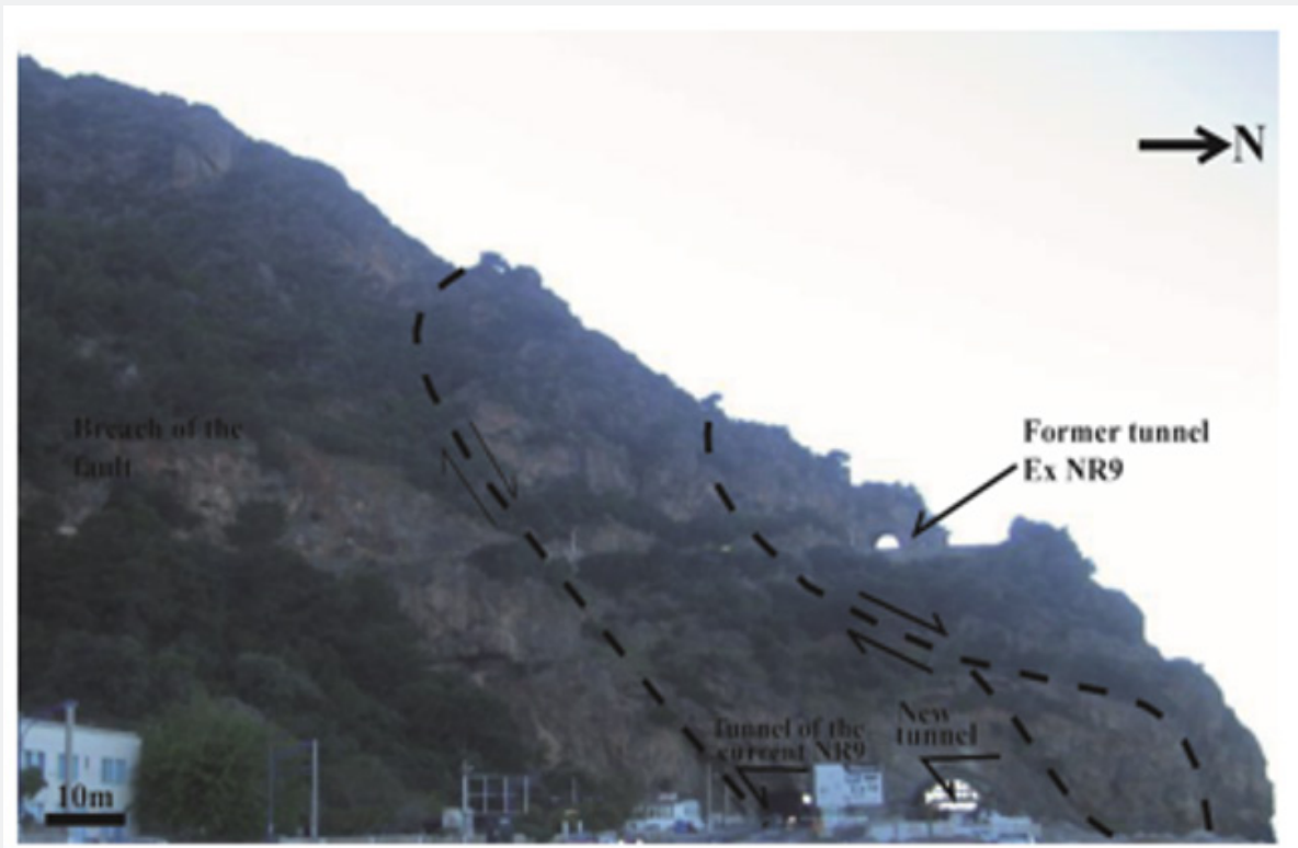
Figure 4: Cutting of the rock massif by normal faults connected to the first family.
