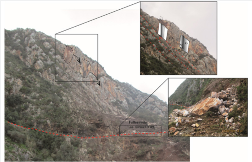
Figure 13: Panoramic photos of dihedrals detached and fallen rocks in the former NR9.
